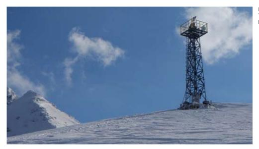
Image 02: The fire detection system is mounted on 20 m high towers
